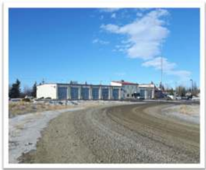
Looking northwest at the tri-services building
